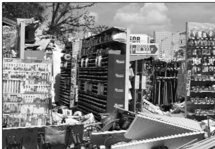
While the walls and roof of Morton's Ace Hardware collapsed, oddly enough a few displays of plastic items remained almost intact.
